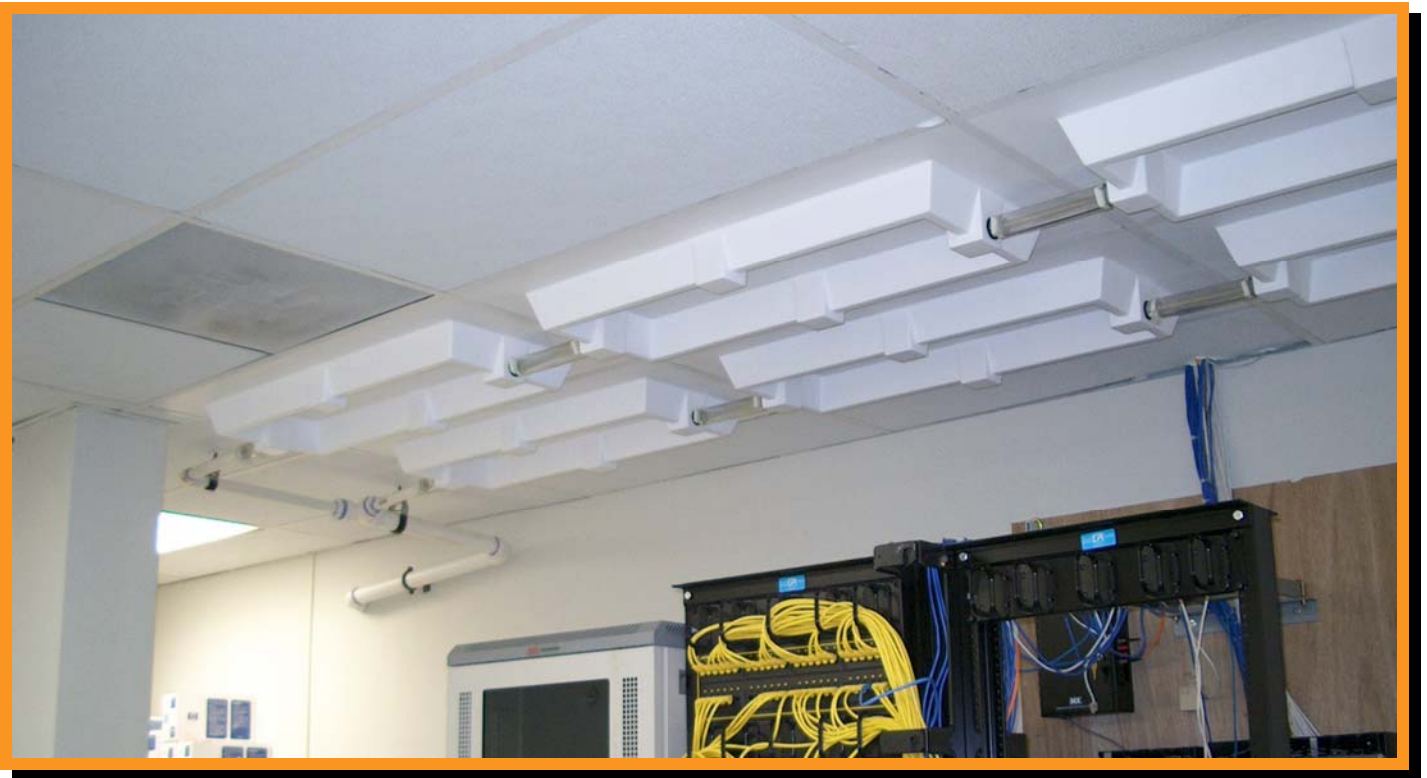
AquaTray ® – 2x4 Leak Barrier Ceiling System (48 square feet) with PVC drain pipe to Janitor's Sink (in next room)
