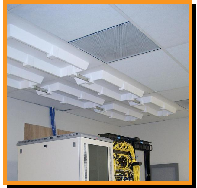
AquaTray® - 2x4 Leak Barrier Ceiling
