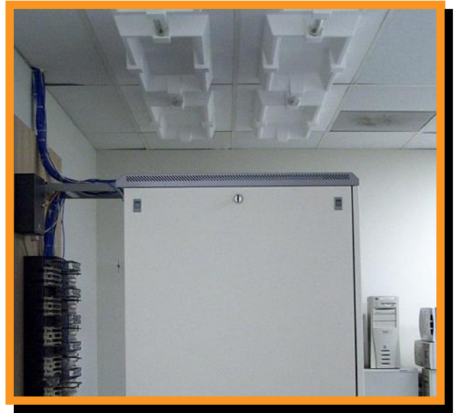
AquaTray® – 2x4 Ceiling Drainage System
